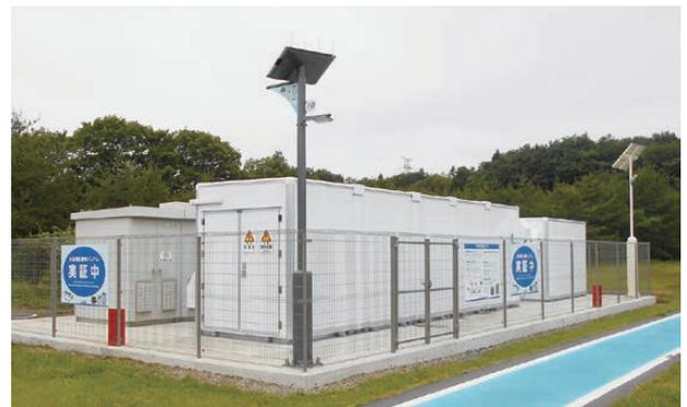
Fig. 1 Appearance of multi-parallel battery energy storage system
