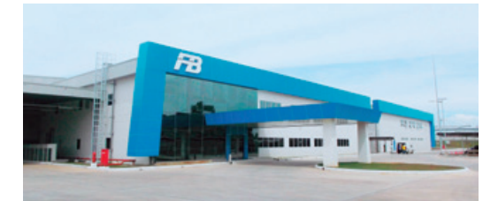
PT. FURUKAWA INDOMOBIL BATTERY MANUFACTURING
