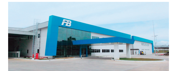
PT. FURUKAWA INDOMOBIL BATTERY MANUFACTURING
