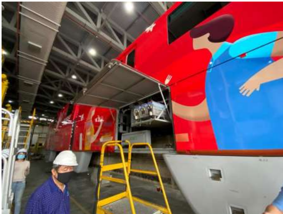
Alkaline storage batteries installed in Sentosa Express in Singapore
