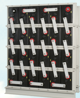
Cycle-use lead-acid batteries
